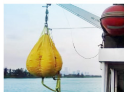
5 Proof Load Testing
